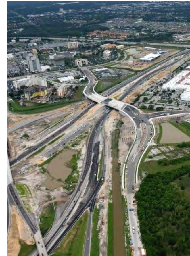
Grand National Drive Flyover
